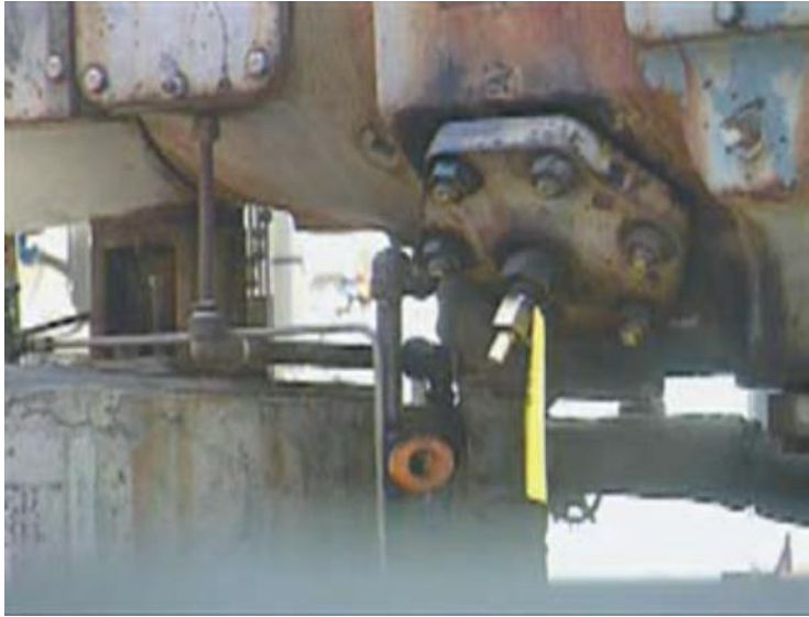
Fugitive emission not obvious within visible light spectrum
