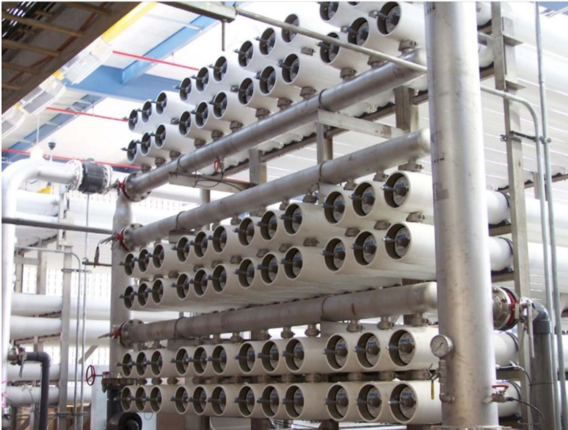
Figure 13. Photo of RO treatment membranes used to desalinate water in El Paso, Texas (Hutchinson, 2007).
