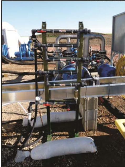
Figure 26. Photograph showing the installation of corrosion test Rack S-2.
