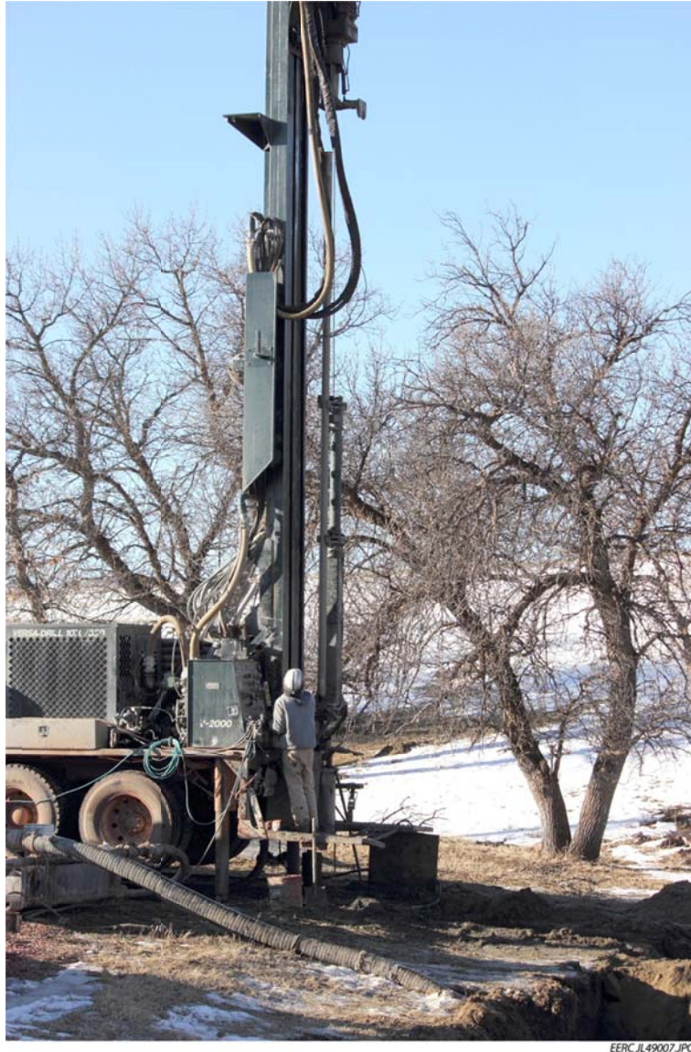
Figure 8. Groundwater-monitoring well drilling 33-12, Bell Creek, Montana (February 2013).
