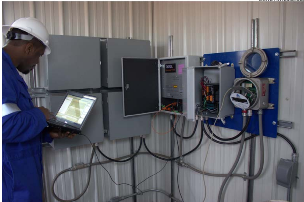
Figure 4. Qorex staff checking the functionality of the fiber optic distributed pressure/temperature data logger (left-most open panel).
