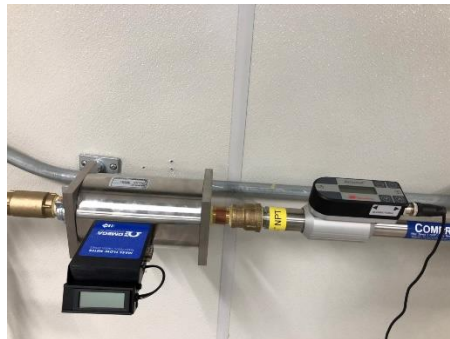
Figure 4 Air flow transmitter
