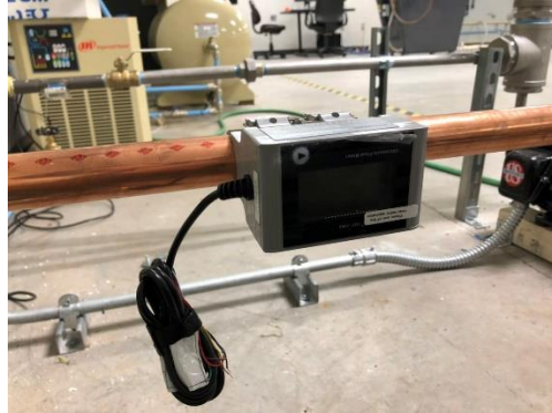
Figure 3 Water flow transmitter
