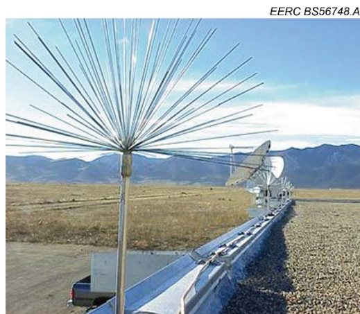
Figure 5. Example of CTS air terminal (source: Lightning Eliminators).
