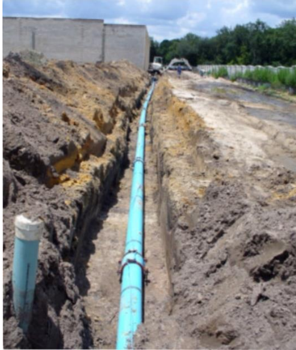
Figure 25. PVC pipeline installation.
