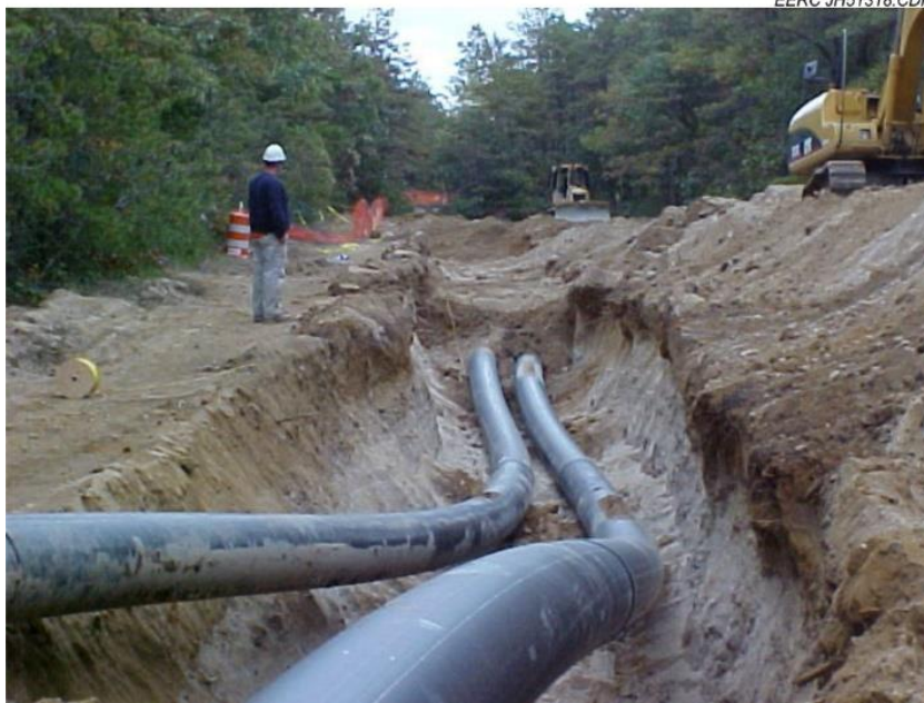
Figure 26. HDPE pipeline installation.
