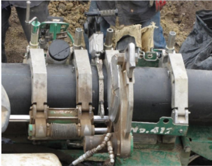
Figure 28. Thermal fusion joint.
