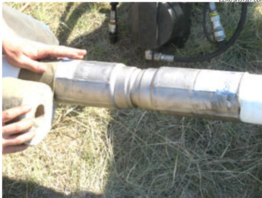
Figure 38. Flexpipe compression fitting.
