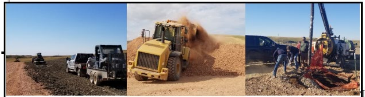
HALITE 1 Wellsite Reclamation.
